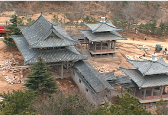
View of the construction underway to expand Chishan Beophwawon
